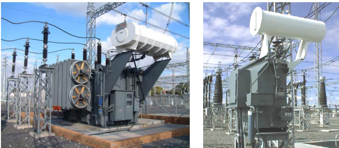
Fig. 1.16: Power transformers
