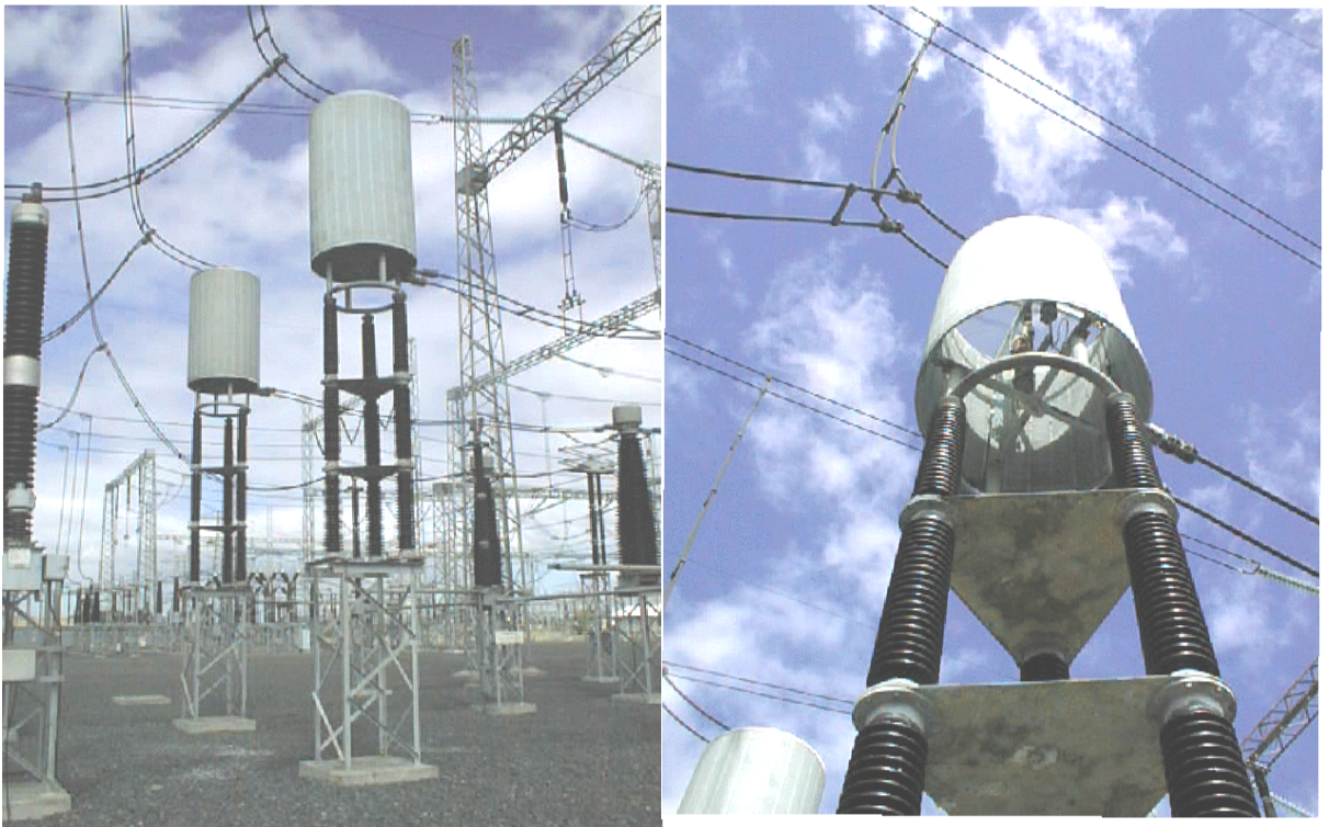
Fig. 1.24: Typical Line Traps
