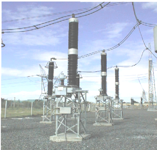
Fig. 1.22 :A high voltage Capacitive Voltage Transformer(CVT)
